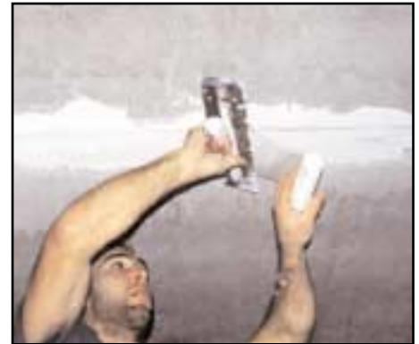
Step 3: Install fiberglass mesh over V-groove.
