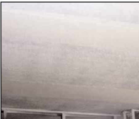
Step 4: Skim coat over mesh, feathering the joint approximately one foot wide or as required.
