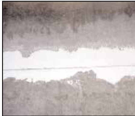
Step 2: Apply second coat over V-groove prior to fiberglass mesh installation.
