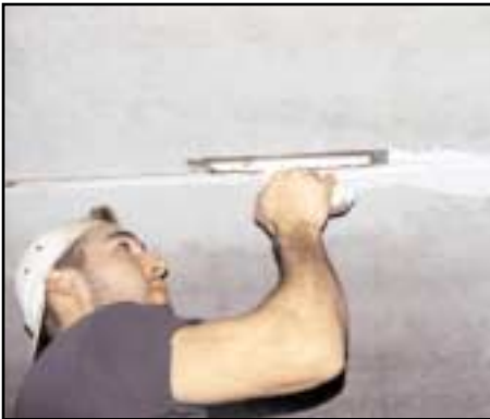
Step 1: Apply joint filler into the V-groove between the Spancrete plank.
