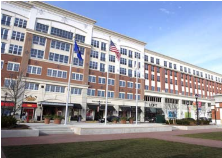
Photo Caption: Spancrete and Corna/Kokosing were recently awarded with Top Project honors for their work on the Bayshore Town Center North Parking Structure, shown here.
